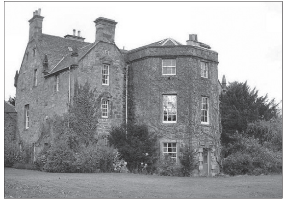
Fig. 2. Baberton House, contemporary photograph showing the semi-octagonal addition by the Anderson family in 1765 between the two projecting wings. (Photograph Muriel Brand 2003.)
