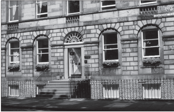
Fig. 2. Formal masonry finishes in Craigeleith sandstone, Abercromby Place. (Photo A. A. McMillan.)
