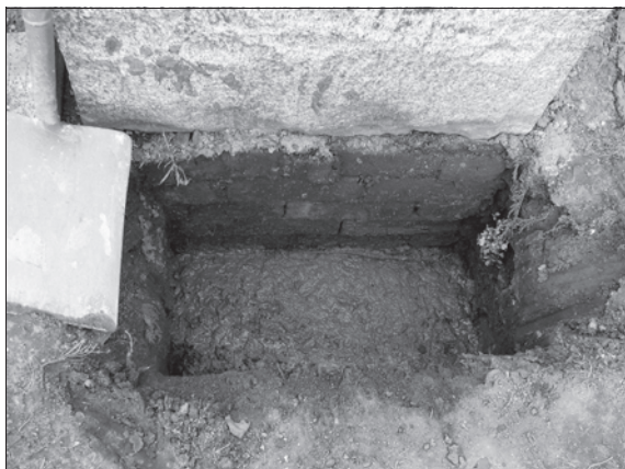
Fig. 6. Previously a brick foundation. (© Alan McKinney.)
