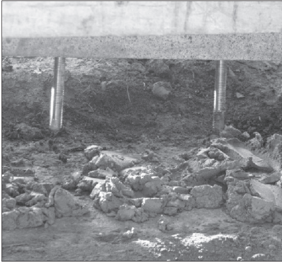
Fig. 9. Soft concrete bed in place. (© Alan McKinney.)
