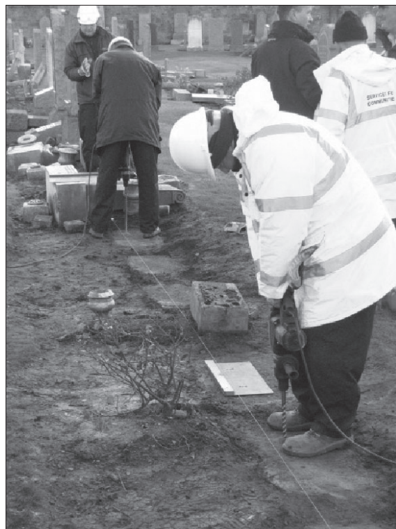
Fig. 7. Using templates, drilling into concrete. (© Alan McKinney.)
