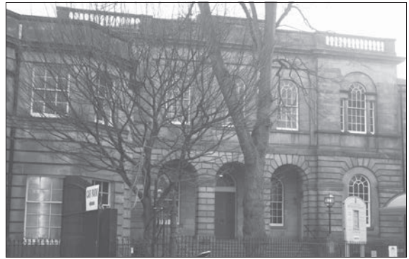
Fig. 5. Nicolson Square Methodist Church with its Georgian façade. (Teri Hopkins-Brown.)
