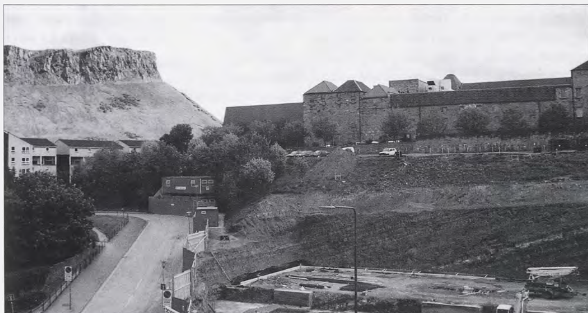
Fig. 8. Photograph taken on 24 May 1996 showing the site of Hutton's house and garden in the clump of trees behind the two cabins of Morrison Construction, Ltd, in Viewcraig Gardens, a late 1960s development. The deep excavation for a car park exposed a 17 metre thick succession of sandstones, siltstones and mudstones of the Cementstone Group. (Photograph by the author.)
