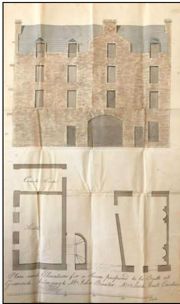
Description: a. Elevation of the tenement and plan of the ground floor. Size: 45.0 x 26.5 cms.
