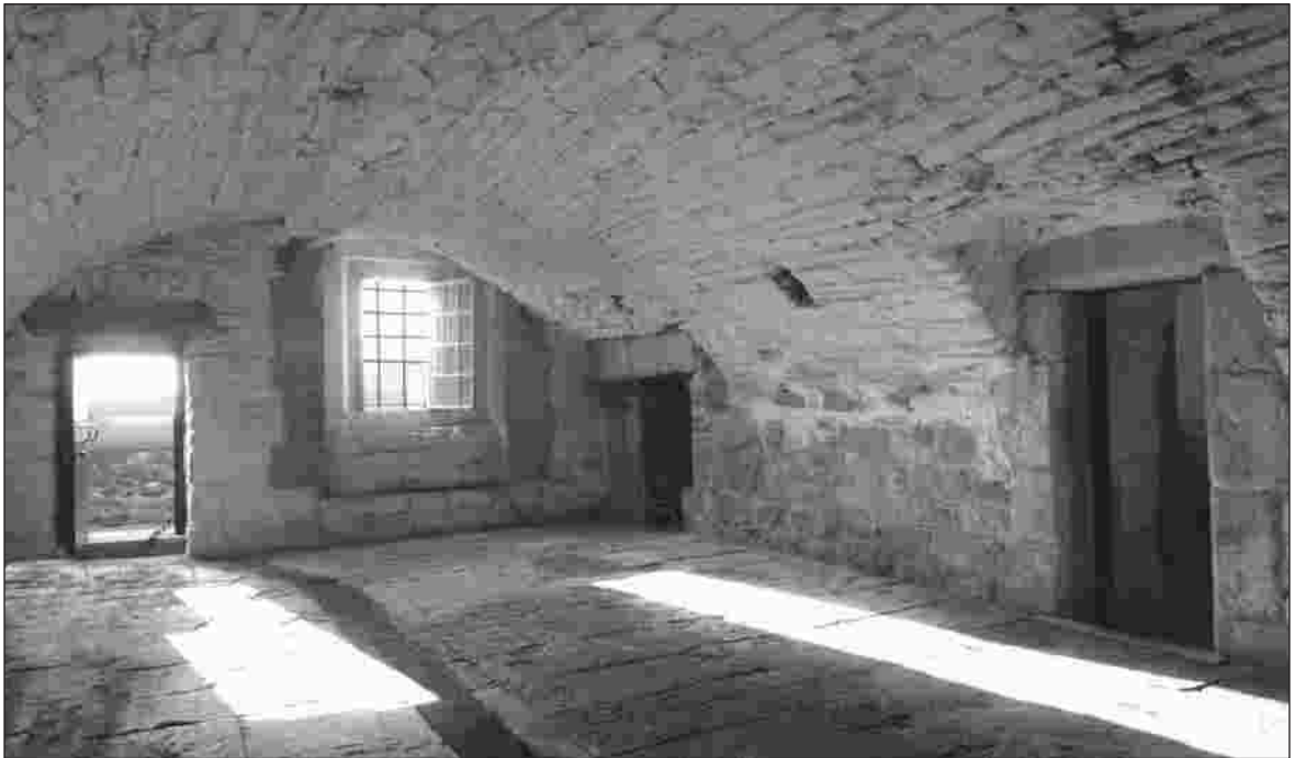
Fig. 4. Vault 5: the stone-flagged floor, narrowed fireplace, door (right) and wall pockets to carry the 'hammer-railing' for the prisoners' hammocks all date from the time the vault was used as a prison of war in the later eighteenth century. ( Historic Scotland. )
