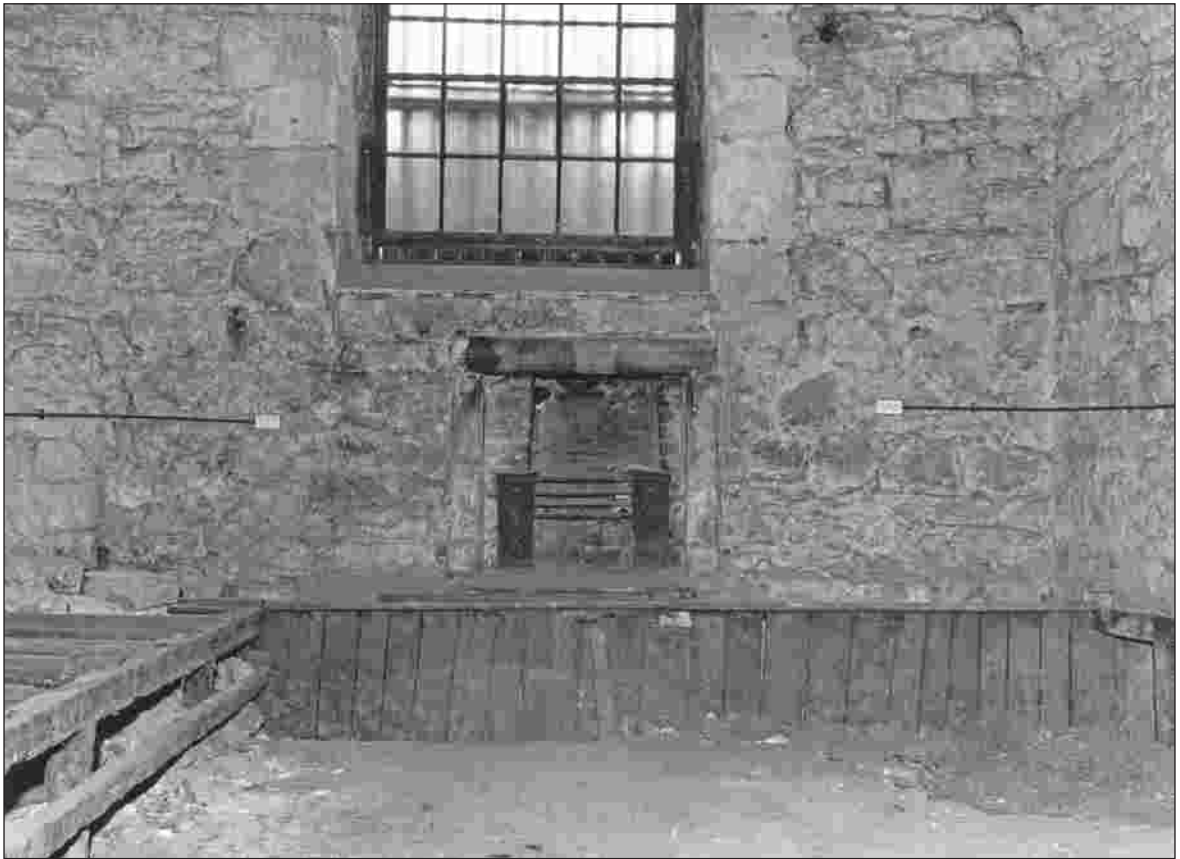
Fig. 9. Vault 3 looking south in 1980. The large window, formed probably in 1778, sits neatly within the fifteenth-century stone jambs. The cast-iron grate bears the royal cipher of George III (1760–1820). ( Historic Scotland. )
