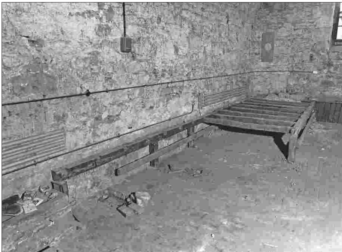
Fig. 10. Vault 3 showing part of the timber framework discovered underneath a raised floor in 1980. The framework, which supported beds, was probably installed in 1778. ( Historic Scotland. )
