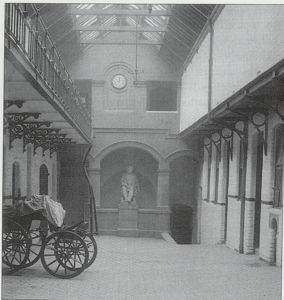
Fig. 23. Photograph, c. 1900, of the north end of the courtyard of the Royal (Dick) Veterinary College, Clyde Street, showing Dick's statue, the doors to the operating room and pharmacy on the right and to the loose boxes and stables on the left. The sloping ramp on the far right leads past the post-mortem room to lower stables and kennels. The balcony on the left leads from the large lecture theatre, via the corridor behind the clock to the dissecting room on the right. (RDSVS.)
