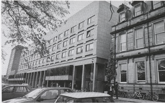
Fig. 17. Photograph of north George Square, 1999. To the right is the former Watson's school, and to the left Walter Ramsay's Pathology Building (1956-62), Phase 1 of the Medical Extension. In the centre is the Hugh Robson Building by Ramsay, with amendments by Basil Spence (1977-80). Phase 3 of the Medical Extension. (Author.)
