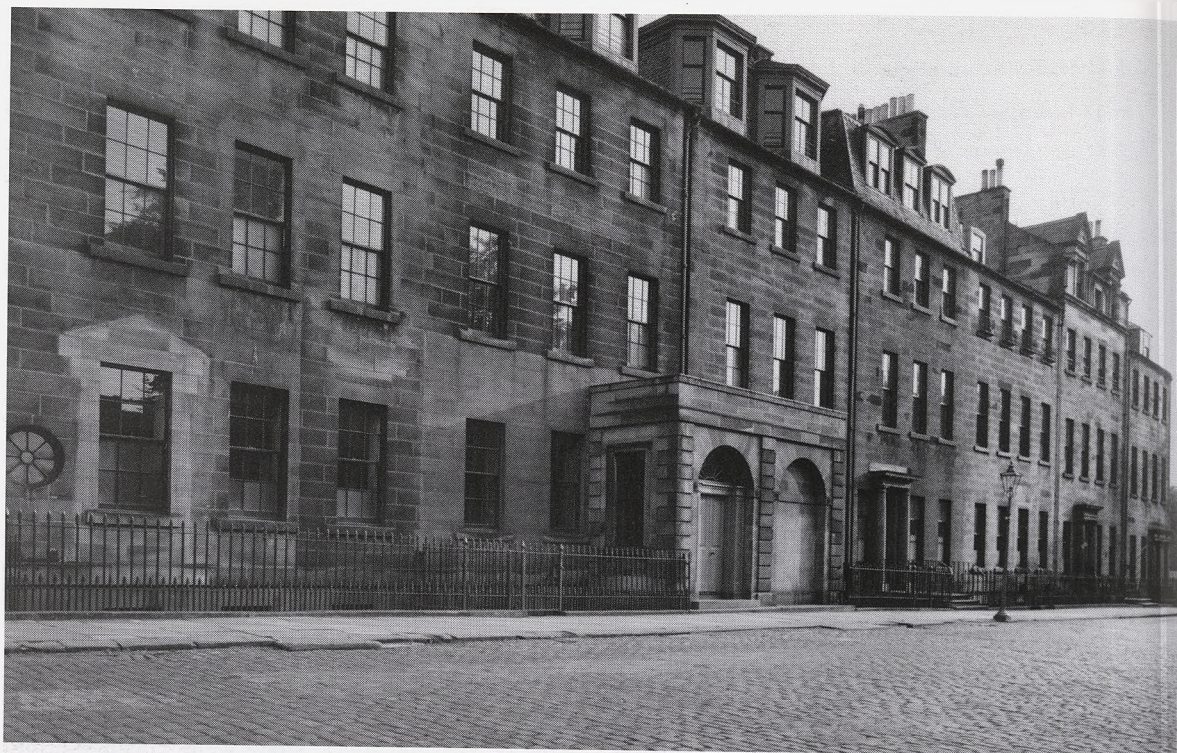
Fig. 4. The west half of the south side of George Square, showing how much the façades of Nos 30–38 had been altered by 1959. On the right, the doorway of No. 32 was removed when it was incorporated into Masson Hall. The doorway to Cowan House (No. 35) shares a porch with No. 34, now blocked. On the left, the portico of No. 36 was removed when the door was converted to a window. All the buildings have also been extended upwards in one way or another. ( EU, Fenton Collection. )
