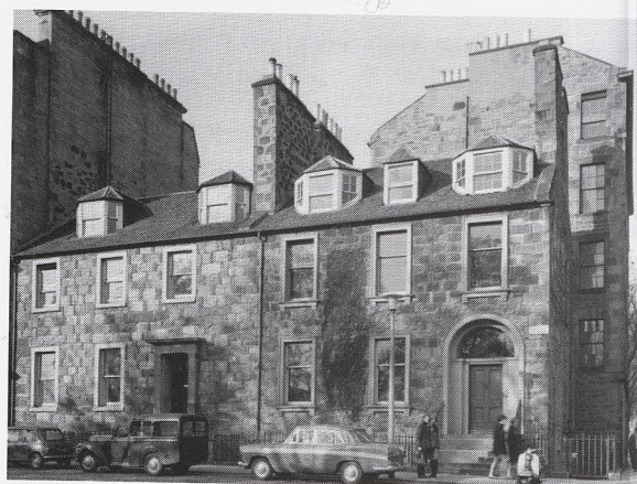
Fig. 2. Nos 1 and 2 George Square, c. 1966. Note the wooden architraves on the windows of No. 1, and the Charles Street tenement to the rear. (Royal Commission on the Ancient and Historical Monuments of Scotland, RCAHMS, No. ED/2338.)
