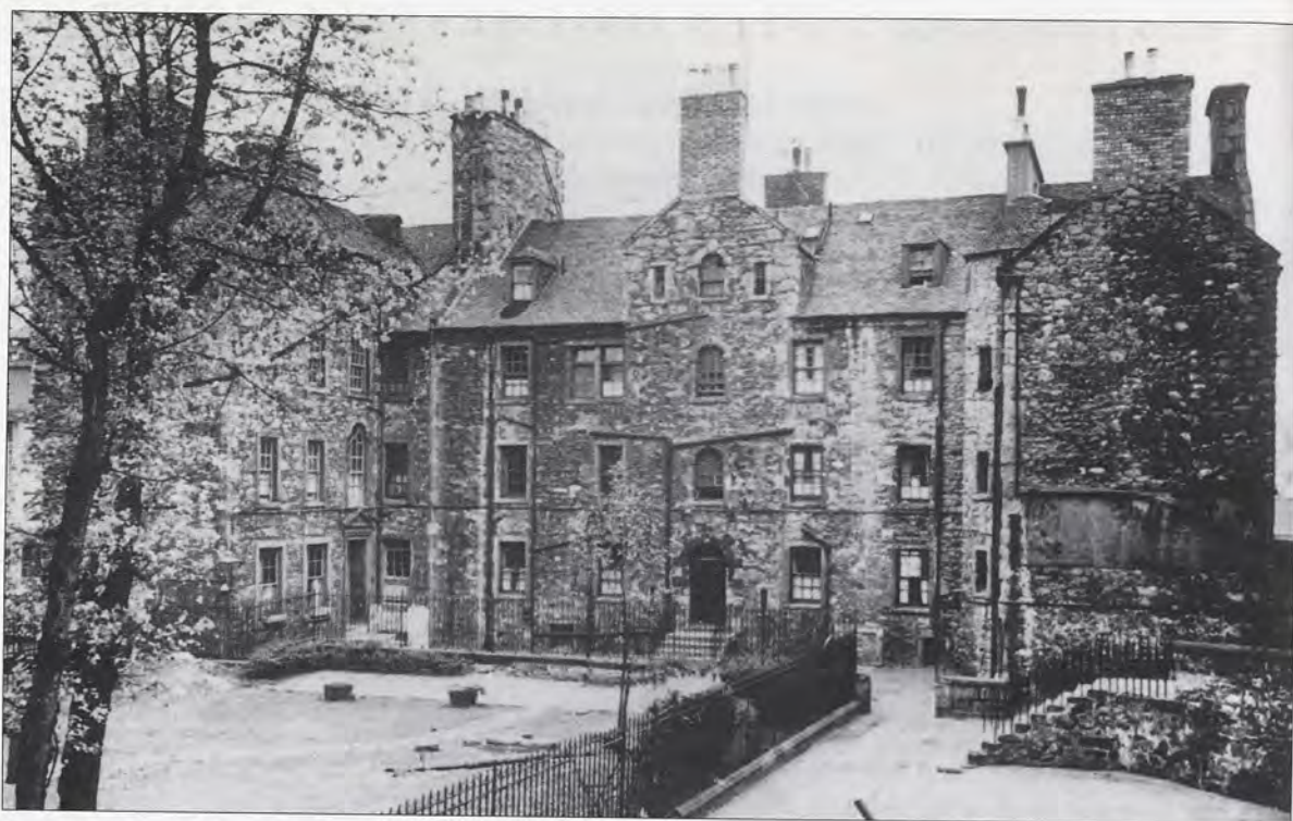
Fig. 1. North front of Chessels Building, including east wing, before refurbishment, 1957. (Photograph courtesy of Hurd Rolland Partnership.)
