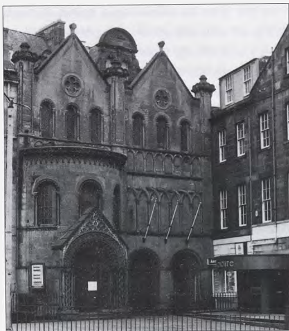
Fig. 1. St Thomas's Episcopal Church, Rutland Place, 1976. ( Royal Commission on the Ancient and Historical Monuments of Scotland. )
