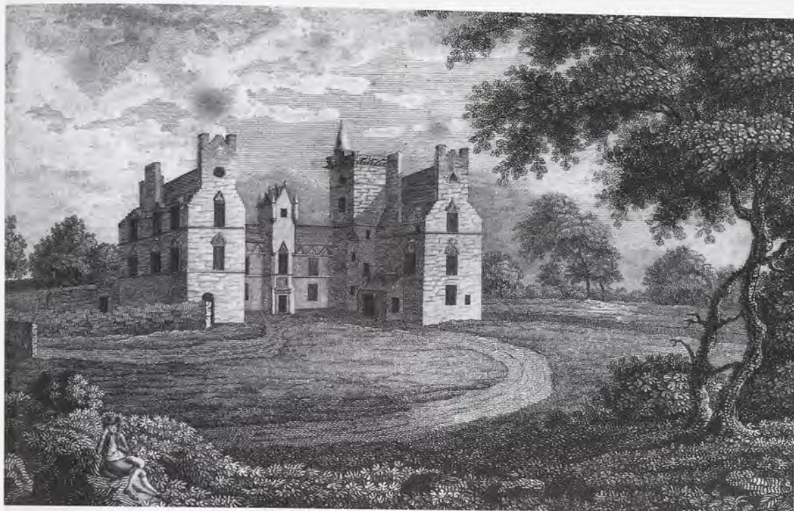
Fig. 5. View from the north east, by J. Dick, c. 1798. Note that the majority of windows in the central range have been blocked (C. McKean; NMRS, A/60739.)
