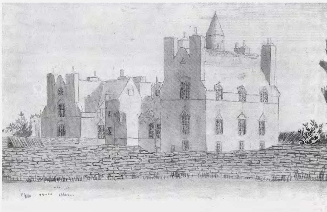
Fig. 4. Wrytes Houses from the north west, drawing by Francis Grose, 1788. ( National Galleries of Scotland , D24.)
